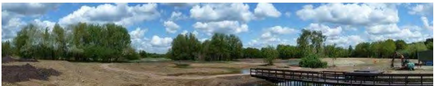
Broadwalk and habitat under construction © WWT Consulting
